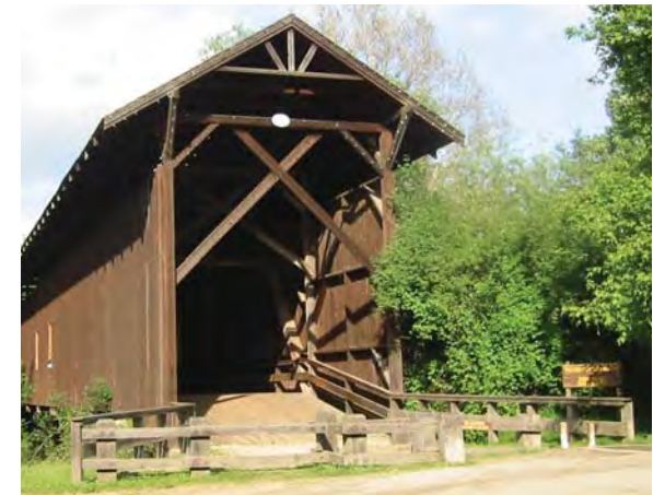
Felton Covered Bridge County Park
